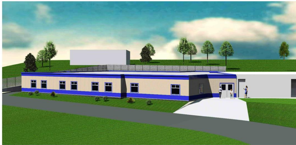
Crescent Park Elementary Modular Addition
